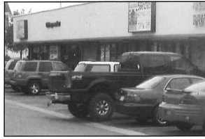
Figure 28 - Inappropriate Wall Sign Combinations on a building face.
