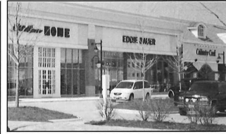
Figure 29 - Appropriate Wall Sign Combinations on a building face.
